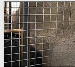
trimming around crooked walls
